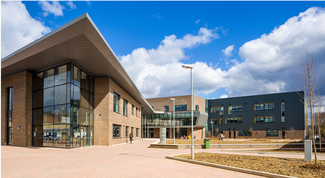
Figure 4 – Morriston Comprehensive (BREEAM Excellent) 2
