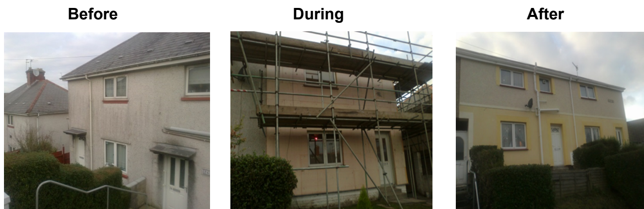
Figure 3 – Typical Enveloping Scheme 1
